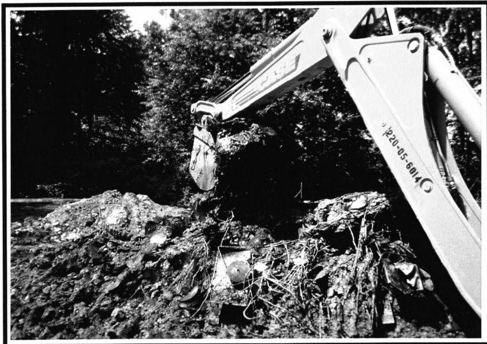
Test Pit TP-96-6
