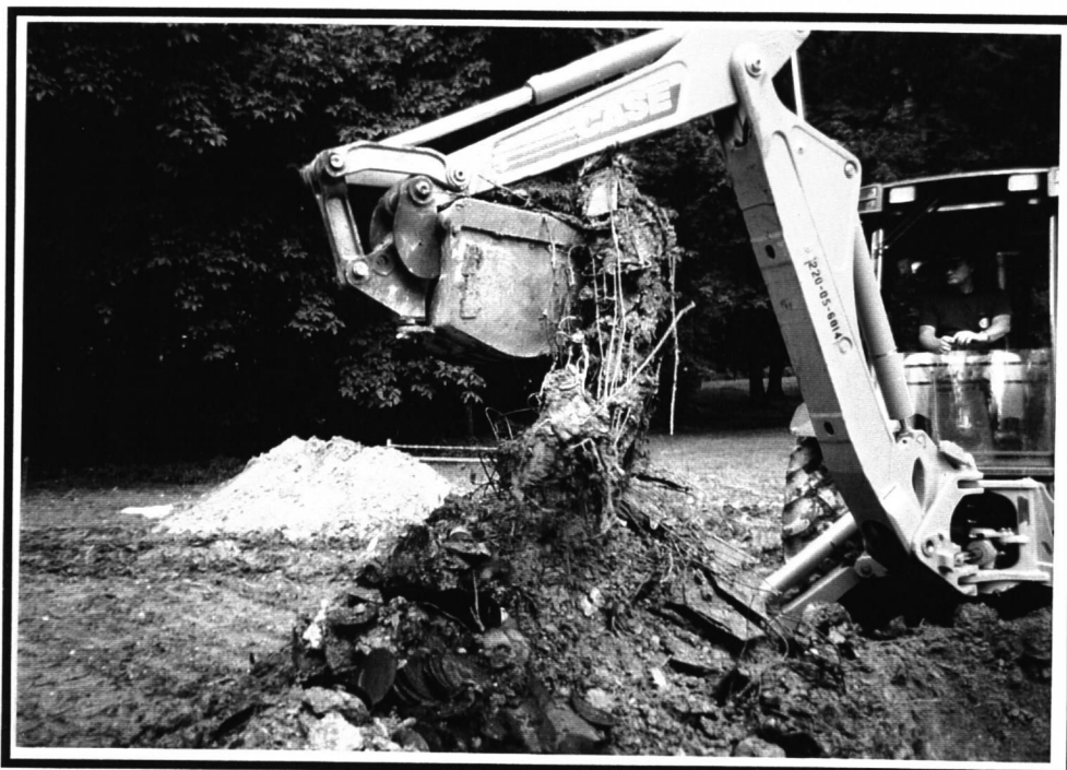
Test Pit TP-96-6
