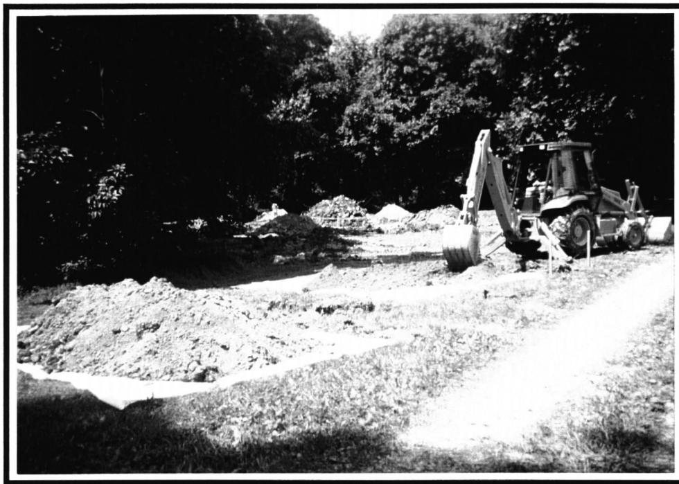
Backfilling Test Pits TP-96-1 and TP-96-2
