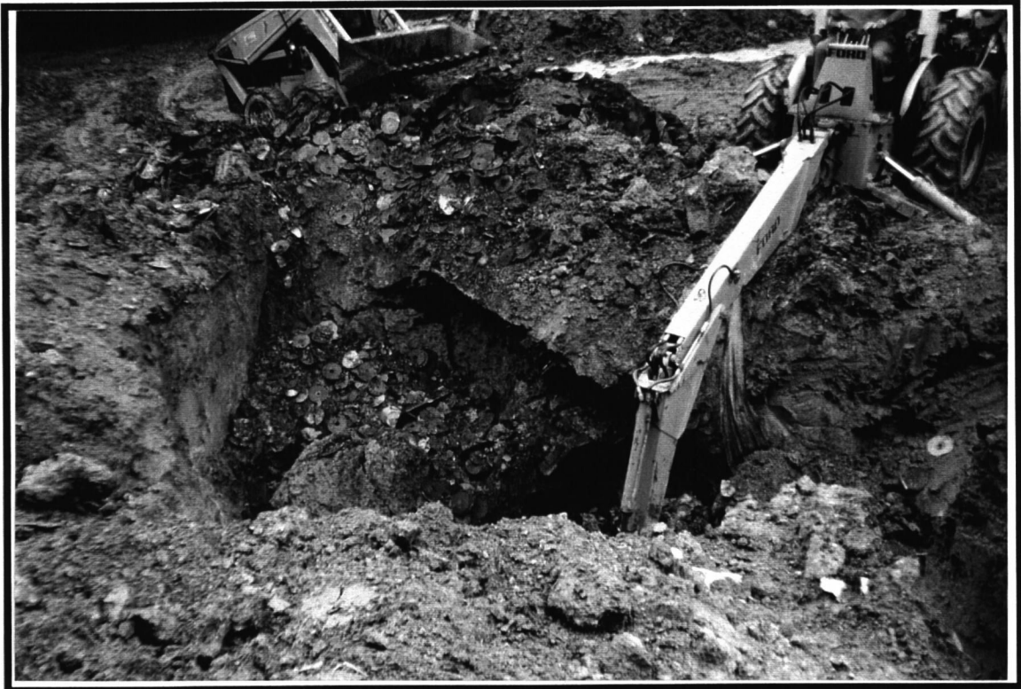
Removal of the remainder of debris
