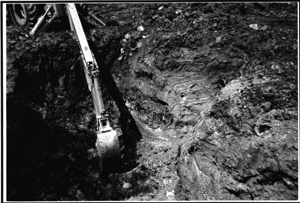
Removal of the remainder of debris
