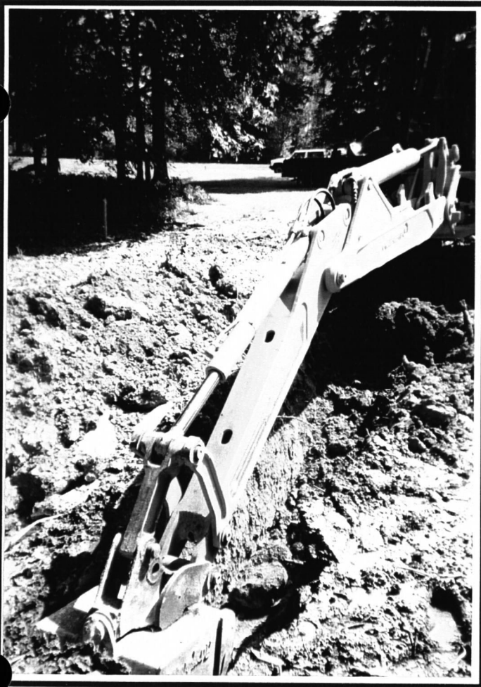
Test Pit TP-96-4
