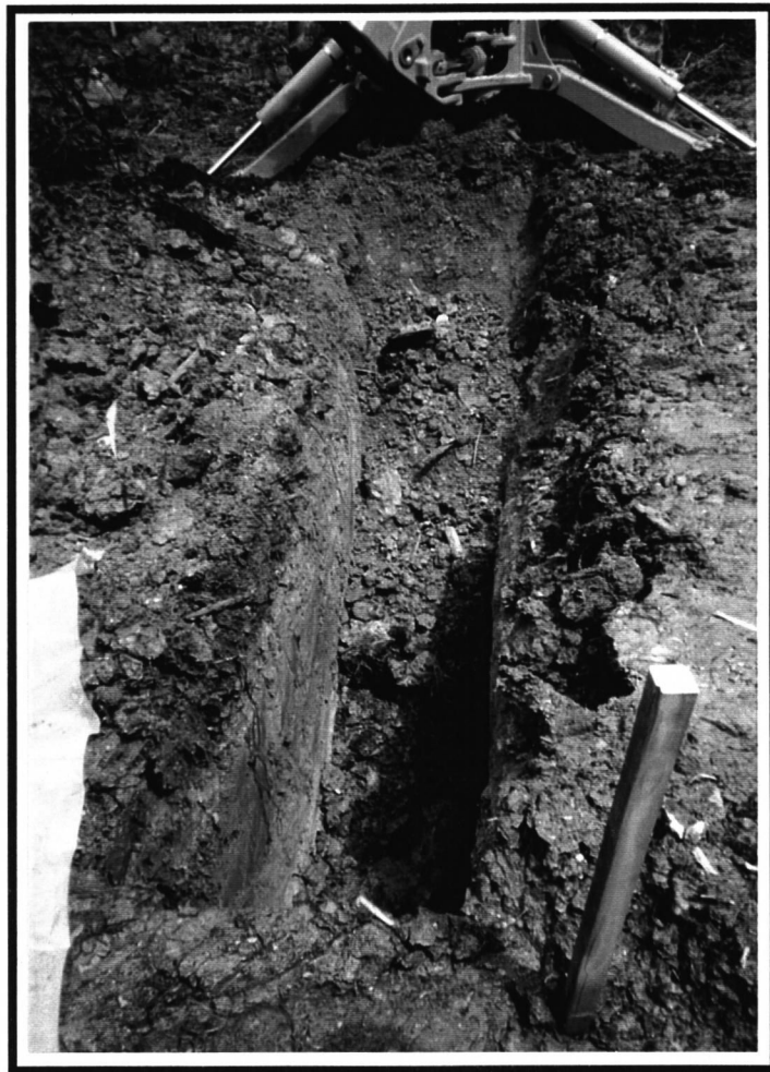
Test Pit TP-96-6
