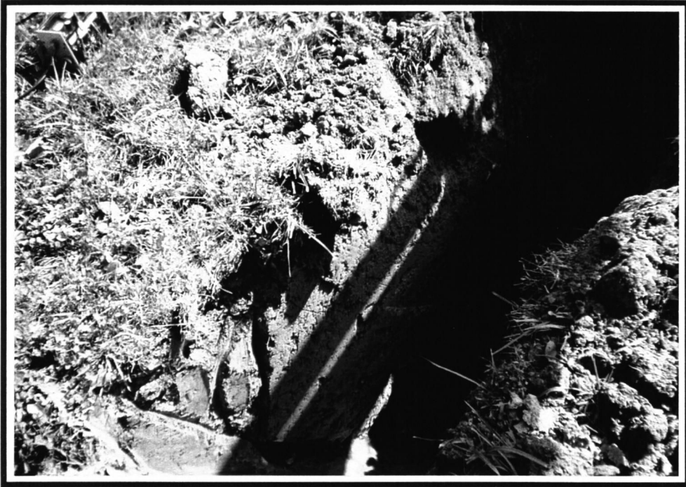
Test Pit TP-96-2
